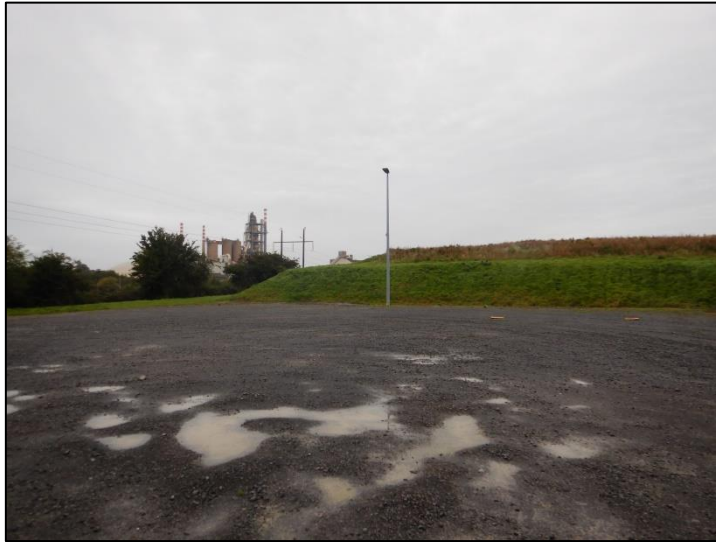
Plate 5: Existing Berm to be increased Area E, looking N
