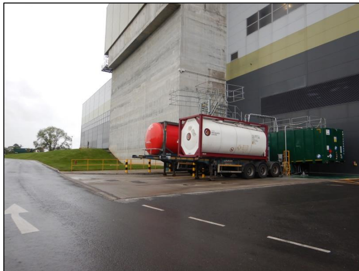
Plate 9: Proposed location for tanker unloading Area 9, looking NW
