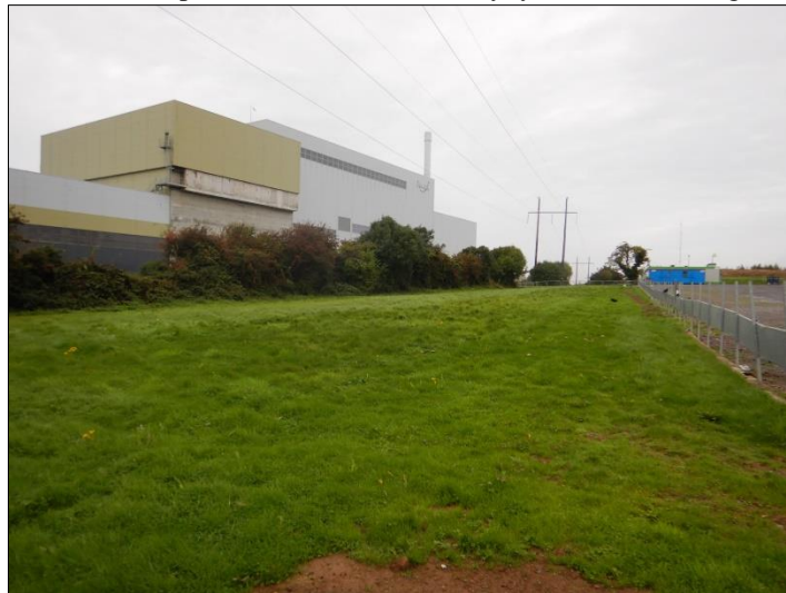
Plate 11: Location for concrete footpath and stairs Area 13 under overhead power line, looking NE
