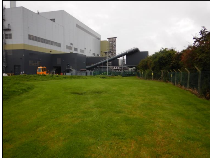
Plate 1: Proposed location for Ash Storage Building Area 1 (B), looking SW
